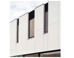
03) - LIGHT CONCRETE LOOK WALL CLADDING
